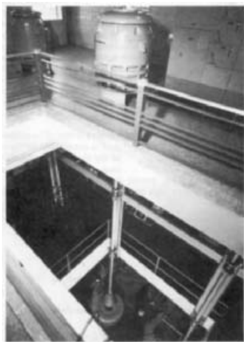
FIGURE 22 Sections of flexible shafts and intermediate guide bearings used to transmit torque from motor located above flood elevation to pump located below ground (Flowserve Corporation)
